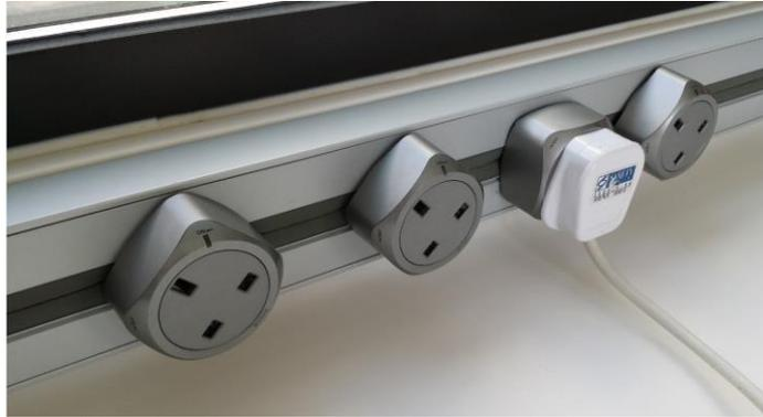
Figure 9: An example of a power track system
