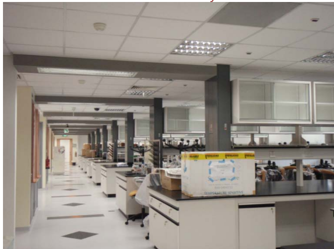
The newly renovated open lab on Level 3.
